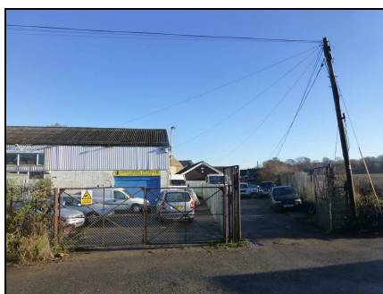
External View – Unit 6
