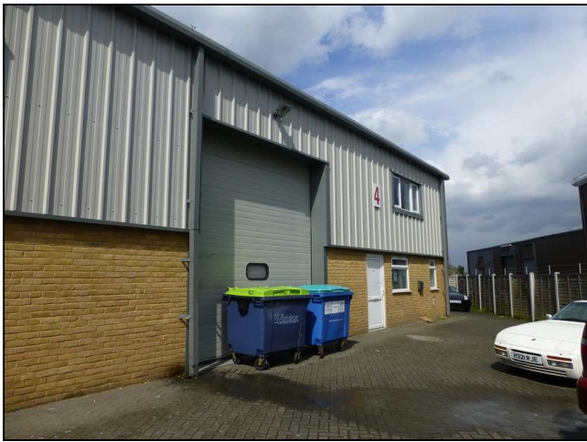
External View of Unit 4
