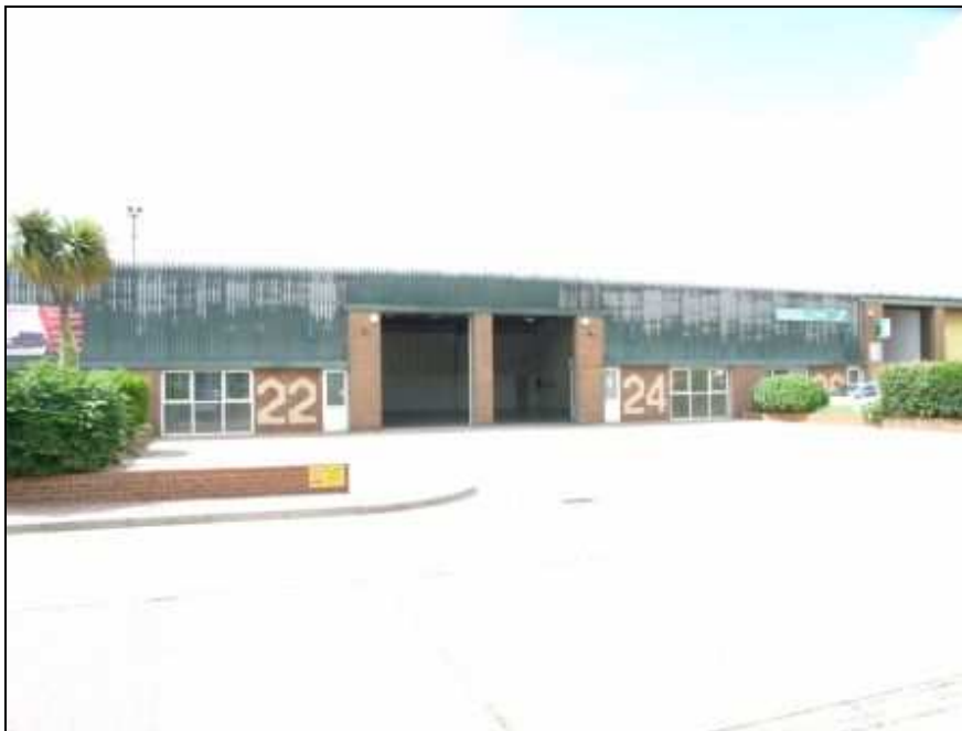
Units 22/24 at Manford Industrial Estate
